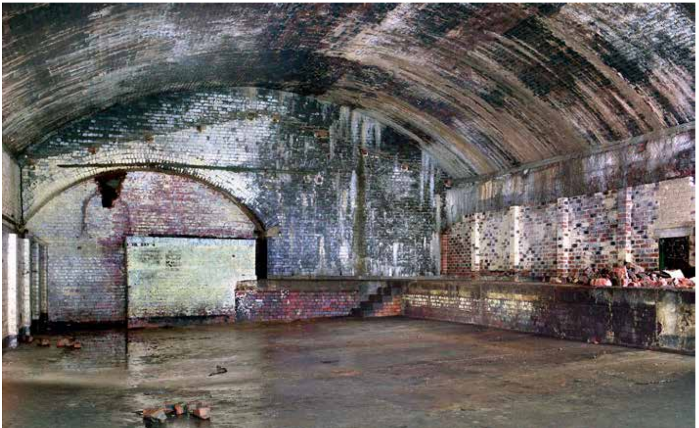
The second trans-shipment dock, with the facing blast wall built into the arch. The passageway set into the tunnel on the right which led to a hoist has been recently blocked off. Photo Nick Catford
